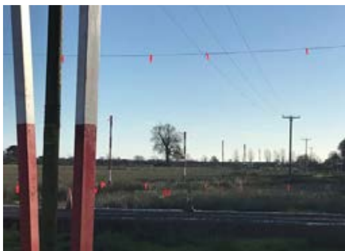
Western power lines removed as part of the wider Lower Otter Restoration Project
